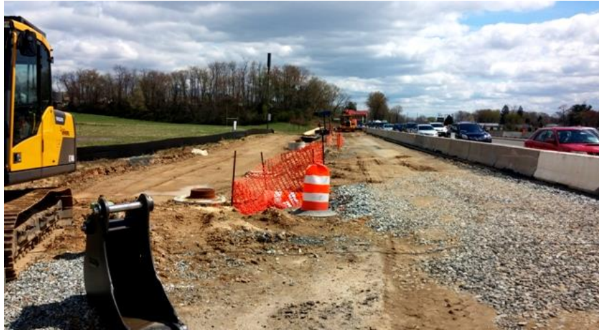
(SHA Photo: Slope grading for MD 22 near Beards Hill Road (MD 132).
